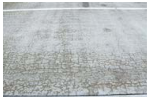
Figure 3. Example of map cracking in unreinforced concrete airfield pavement.
